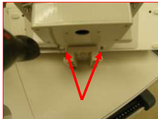
Figure 37. Tightening back screws
