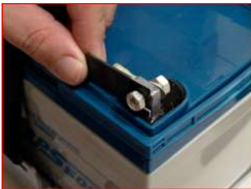
Figure 52. Placing Thermal Sensor
